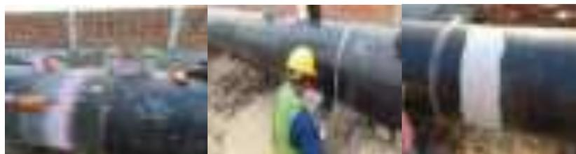
**Gambar 64.** *Penetran Test, Wrapping, Coating*
