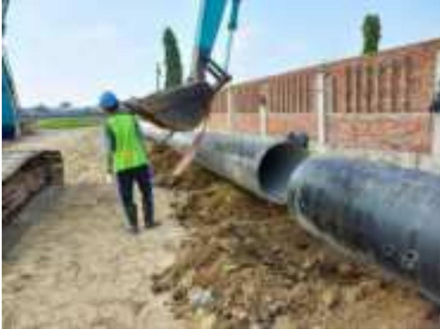
**Gambar 62.** *Fit-Up Pipa Steel*
