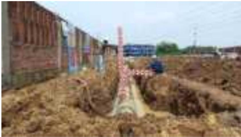
**Gambar 65.** *Penetran Test, Wrapping, Coating*
