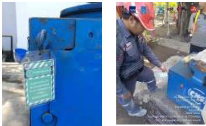
Gambar 11. Contoh Penerapan LOTO diproyek CWI-01 ITS
