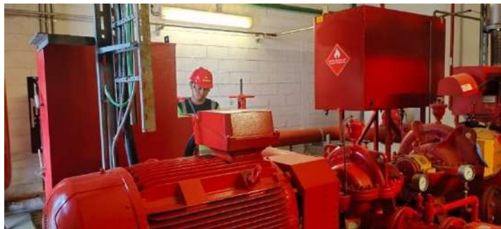
Gambar 3. 6 Inspeksi Pump House
