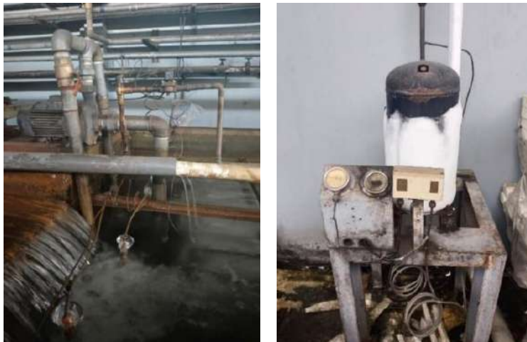
Gambar 26. Bak Air Dingin ( Cooler ) : (a) bak air dingin (b) Cooler
